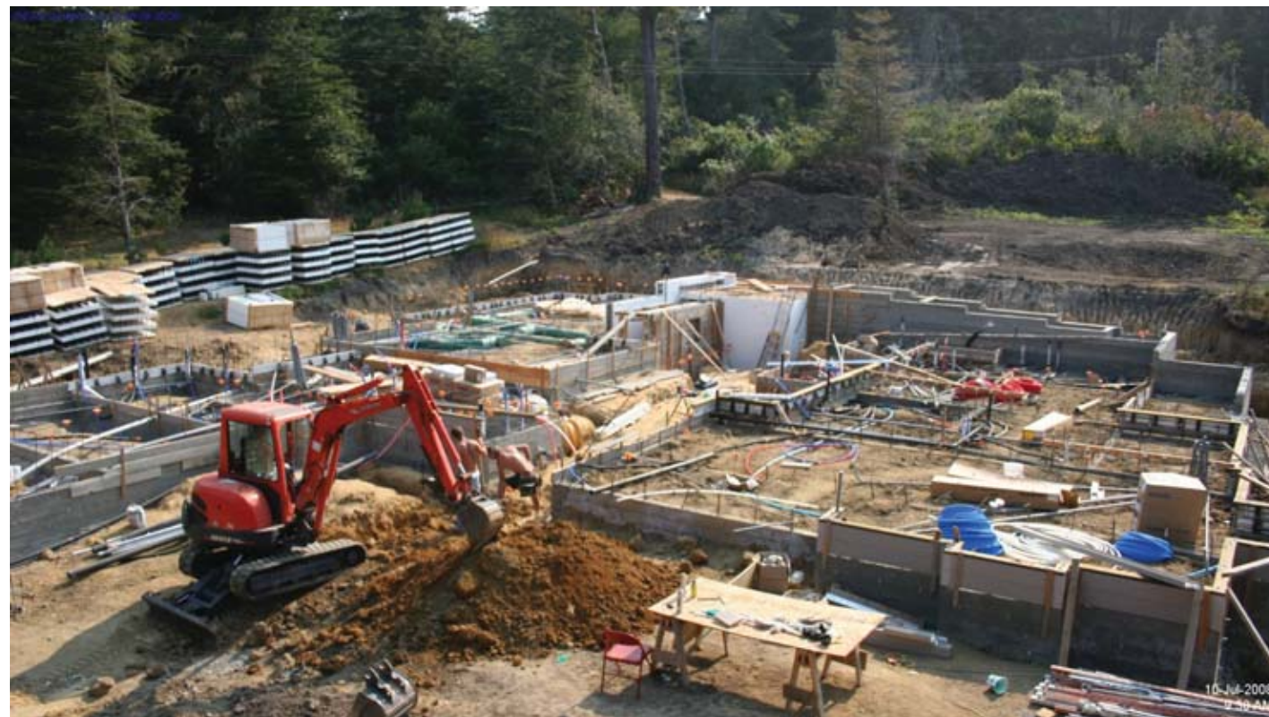
iBeam Time-Lapse Pro Construction Camera Perspective
