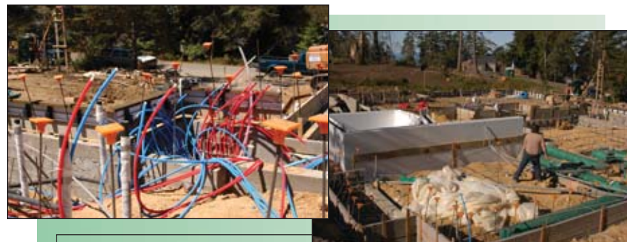
Clockwise: Uponor Plumbing, Electrical Conduit, Amvic ICF Underground Wine Cellar, Energy Edge
