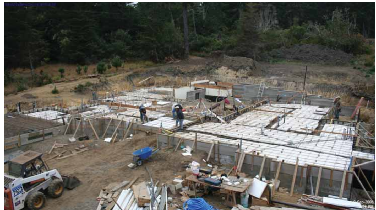
iBeam Time-Lapse Pro Construction Camera Perspective 2008-09-09
