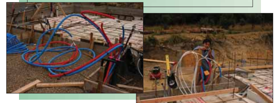
Above: Uponor AQUAPEX Radiant Tubing, Spunstrand Saddle Vents Below: Uponor Radiant Send & Return
