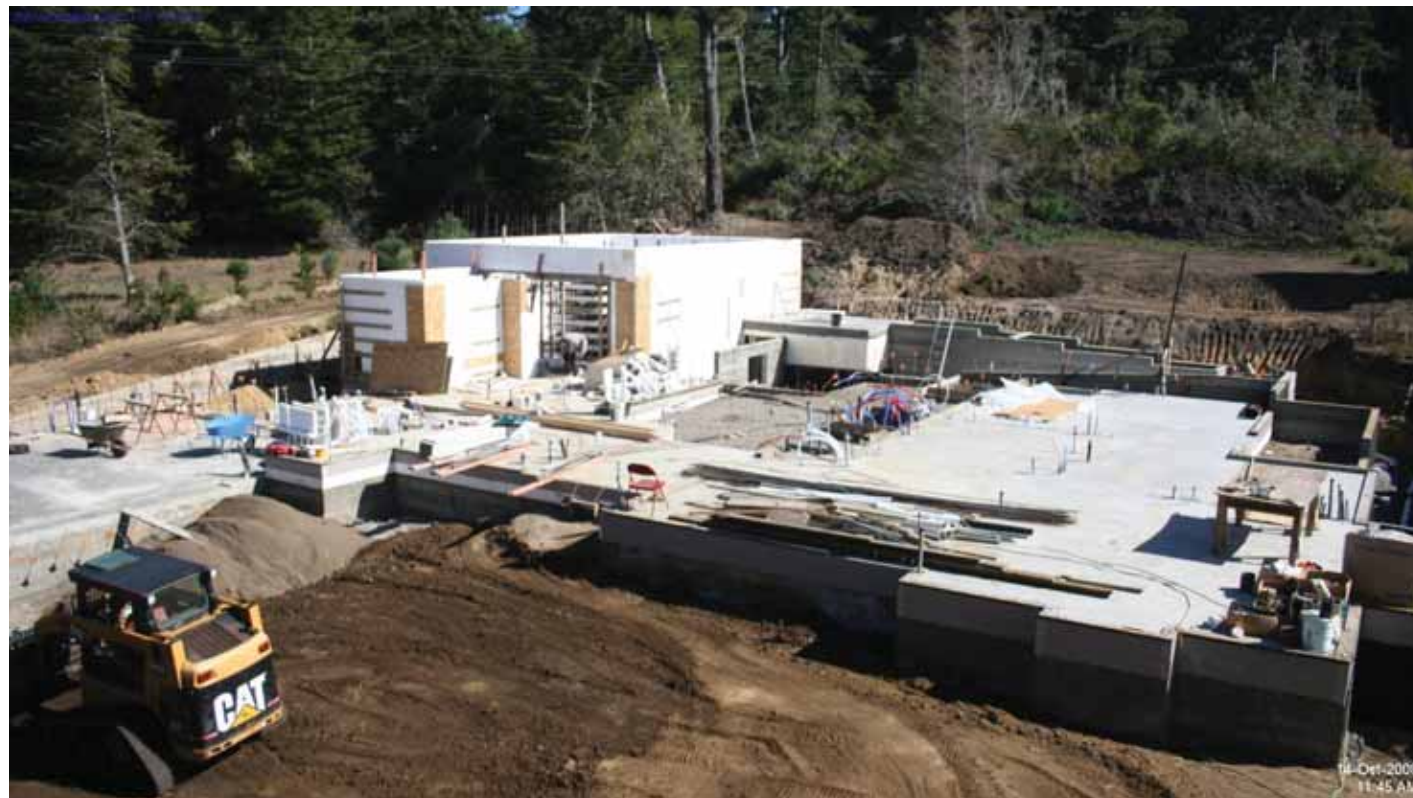
iBeam Time-Lapse Pro Construction Camera Perspective 2008-10-14
