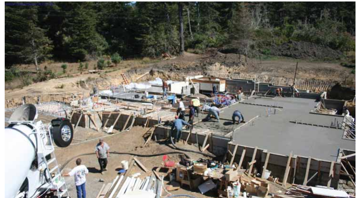
iBeam Time-Lapse Pro Construction Camera Perspective 2008-09-22
