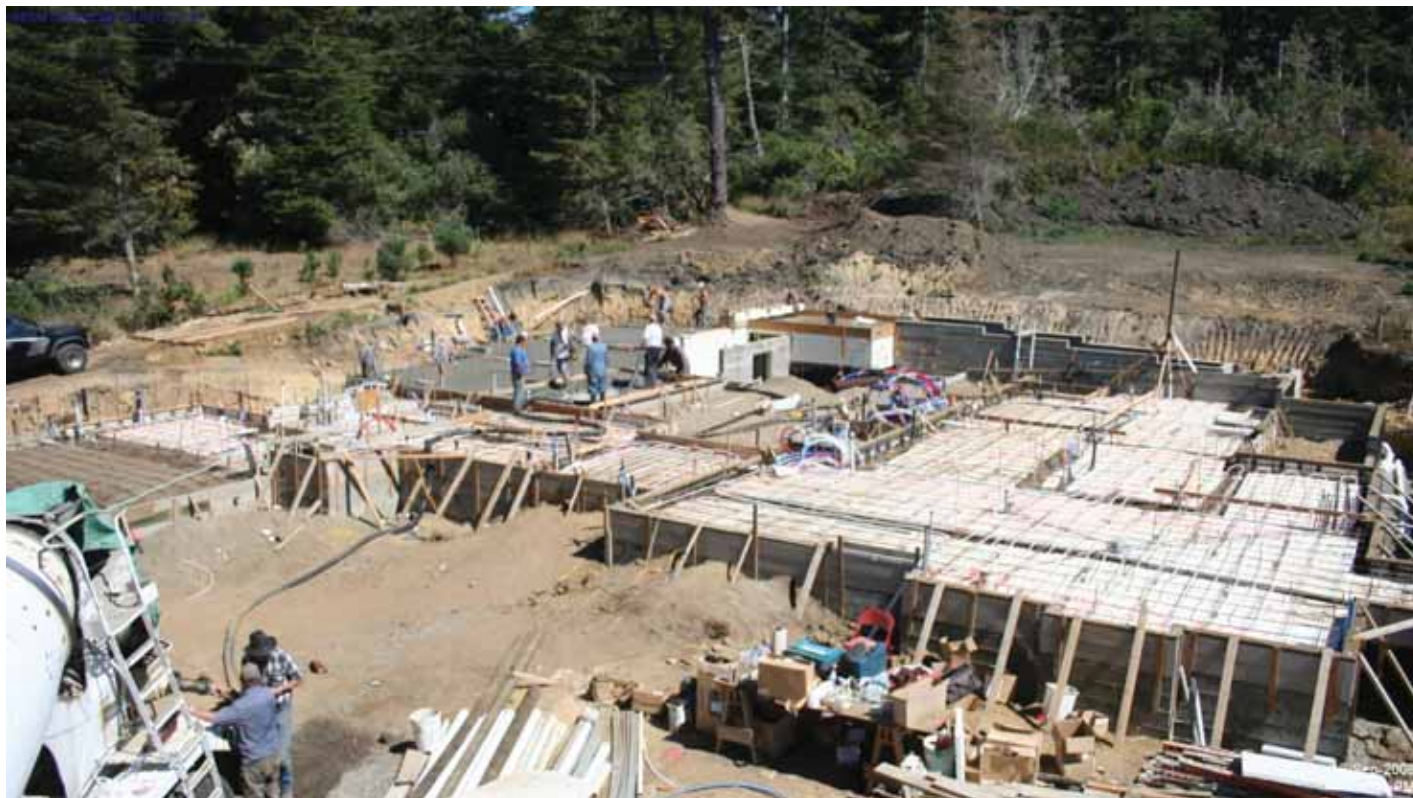
iBeam Time-Lapse Pro Construction Camera Perspective 2008-09-18
