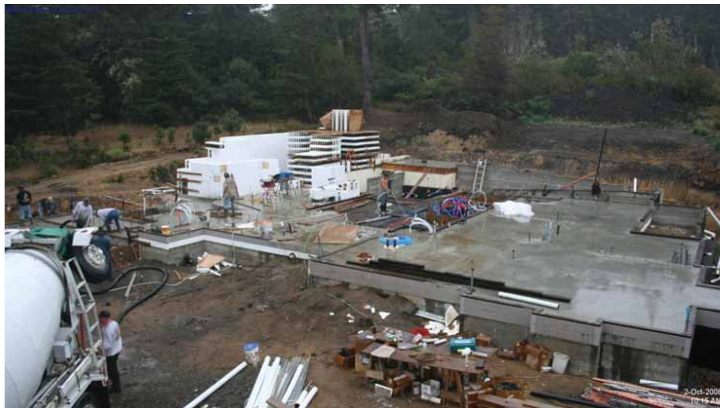
iBeam Time-Lapse Pro Construction Camera Perspective 2008-10-02
