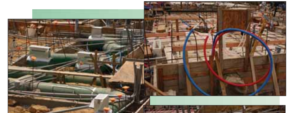
Clockwise: Uponor Radiant Send & Return, Spunstrand Saddle Vents, Uponor AQUAPEX Radiant Tubing
