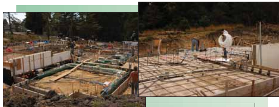
Clockwise: Infrastructure Overview, Uponor AQUAPEX Radiant Tubing, Wine Cellar, Uponor Radiant Send & Return
