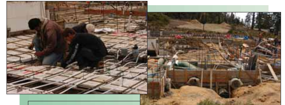
Above: Uponor AQUAPEX Radiant Tubing, Spunstrand Saddle Vents Below: Uponor Radiant Send & Return
