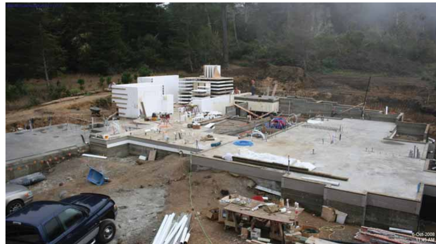
iBeam Time-Lapse Pro Construction Camera Perspective 2008-10-06
